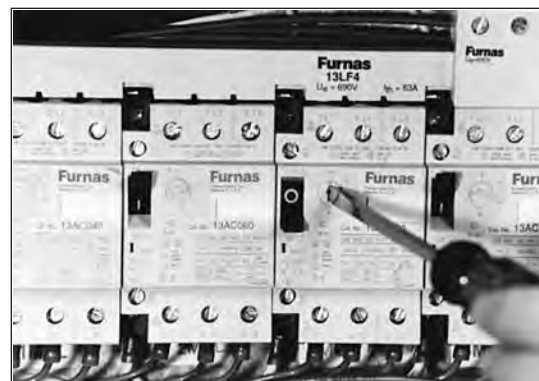
Figure 3 Motor Overloads
