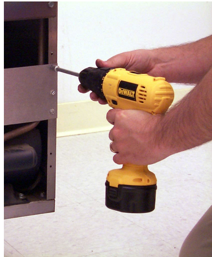
Removing gas manifold shield.
