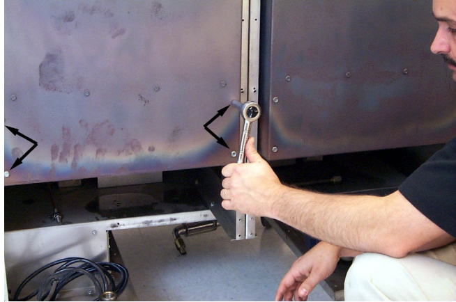
Removing bolts (arrows) securing flue to cookpot.
