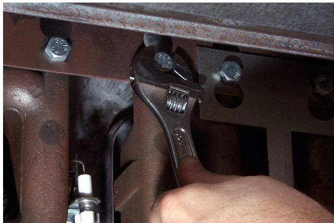
Loosening burner bolts prior to burner removal.
