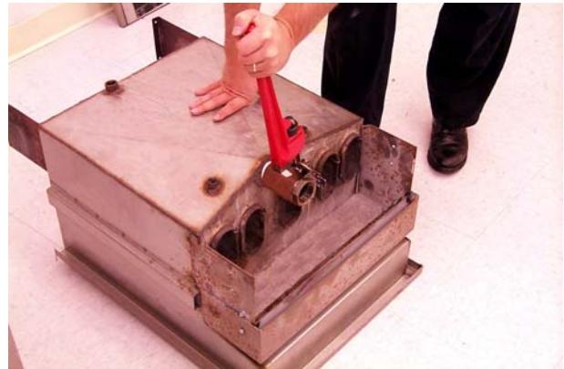
Removing drain valve from frypot.
