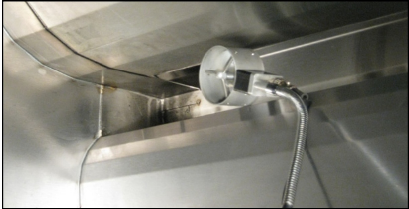
Figure 5-3-1 Sensing Head at Air Inlet Slot
