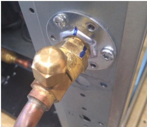
Picture 5: Turn 60° that correspond to one face of the hexagon
