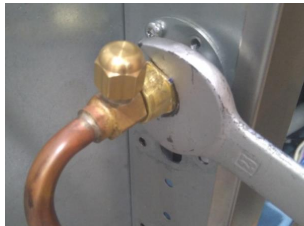
Picture 4: Tighten with a fixed wrench clockwise
