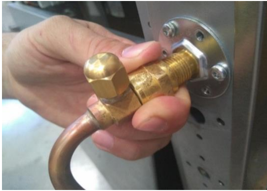
Picture 2: Thread the couplings by hand
