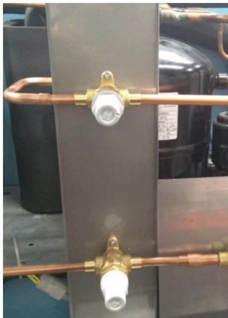
Picture 6: Cut-off valves inside the ice machine
