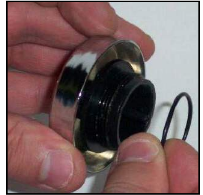
Replacing the O-ring
