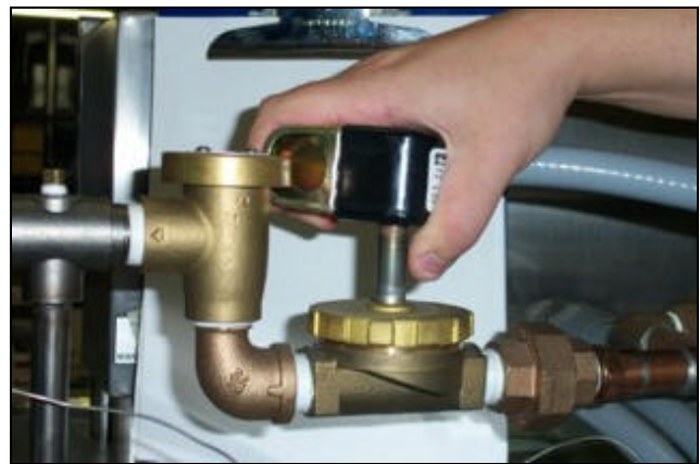
Removing the coil
