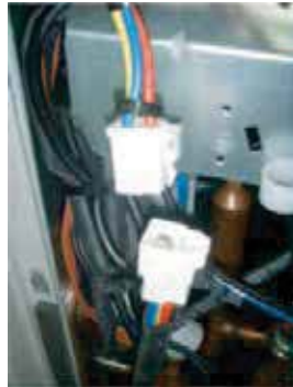
Figure 50: ARUN060GSS4 and ARUB060GSS4 Error No. 29 Compressor Terminal and Wiring Connections.
