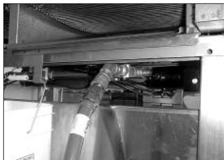
N2500 Equipment Side Gas Connection
