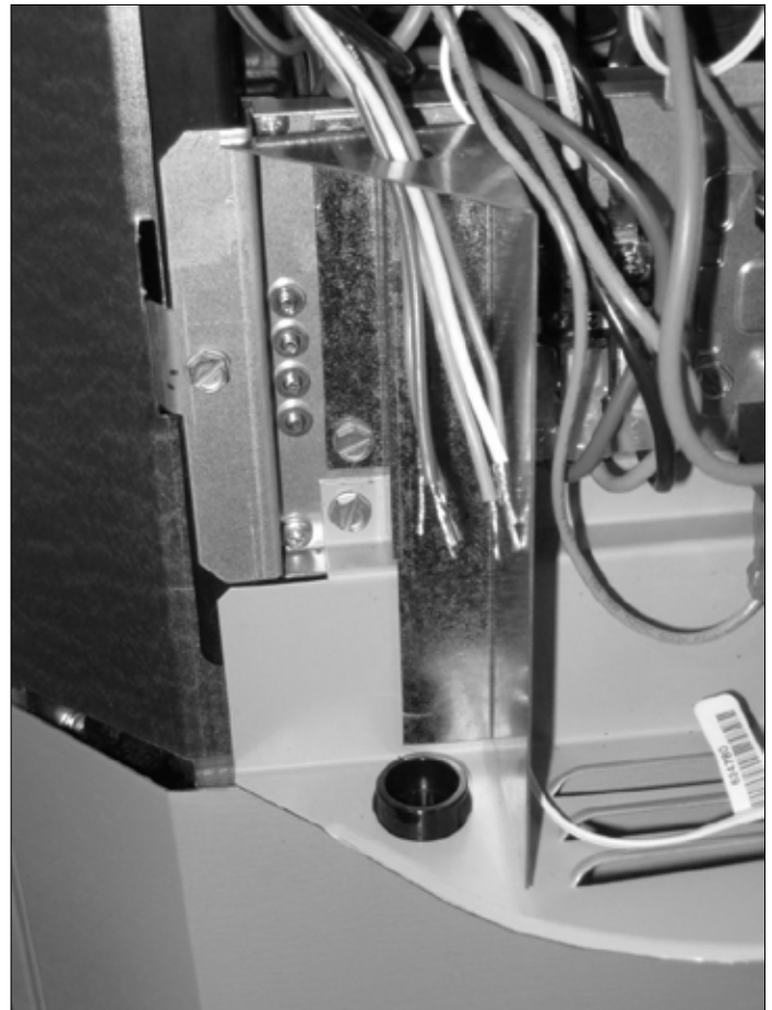
Figure 4. Low Voltage Compartment for Control Wiring
