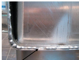
SEALANT APPLIED TO INTERIOR SURFACE OF TRIM PLATE
