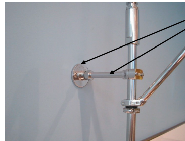
Cut the riser support rods to the proper length and attach flanges to the wall
