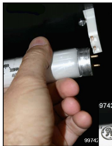
View of Removal / Install of Standard Fluorescent Light Fixtures
