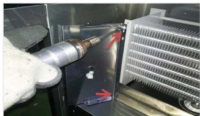
L . Disconnect the harness sensor.
