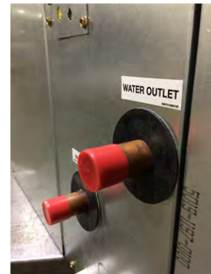
Figure 31. Clean panel before installing grommets
