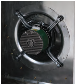
Figure 75. Blower coil with Trane ECM motor
