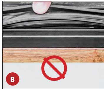
Fig. 12. Pull the side of the gasket to check its installation.
