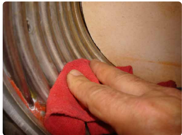
Figure 152 Cleaning the heat exchanger
