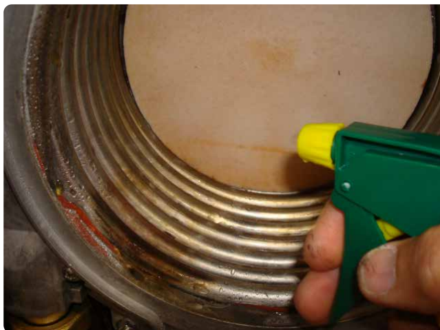
Figure 150 Cleaning the heat exchanger
