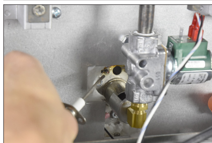
3b Pulling Igniter
